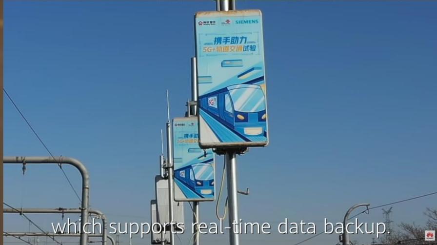
These are 5G leaky cables
